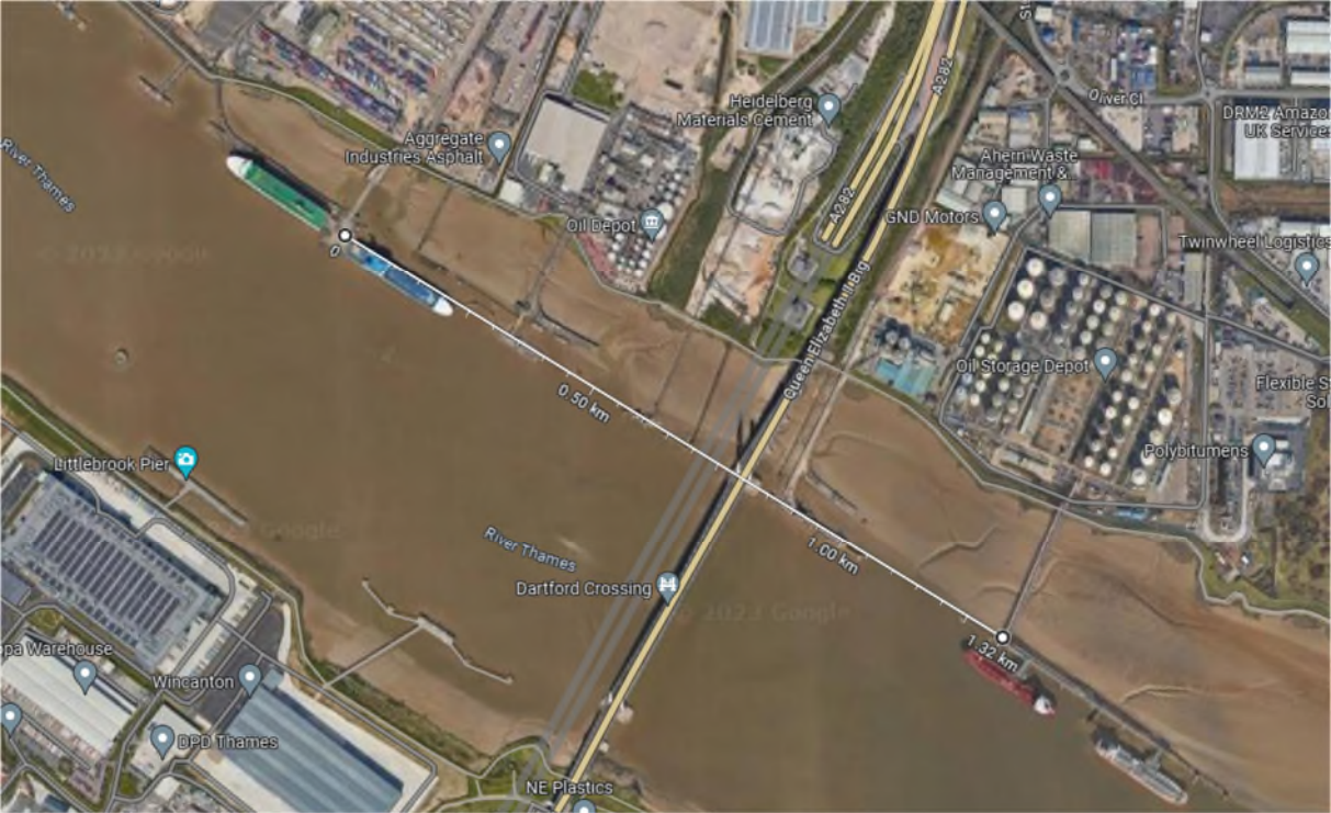
Figure 1: Distance between petrochemical apparatus and the CLdN Ro-Ro facility at Purfleet
